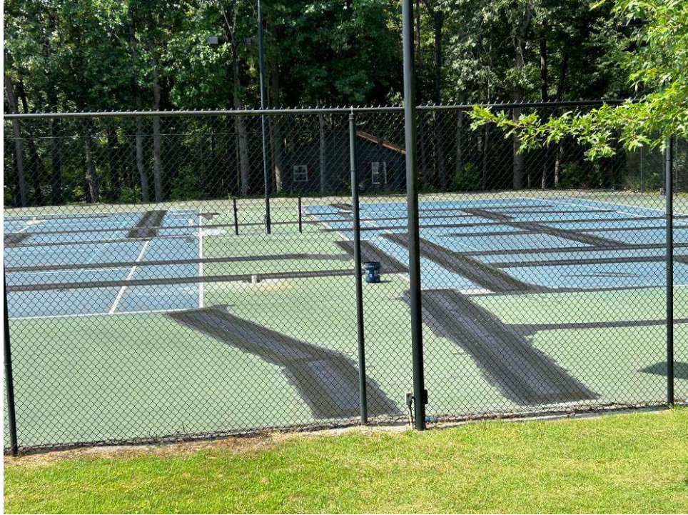
13. View of tennis court being resurfaced.
