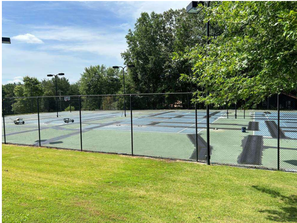
12. View of tennis court being resurfaced.
