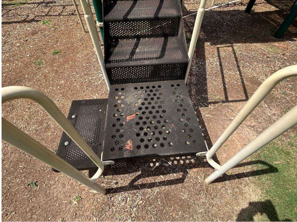
15. View of cracked playground equipment piece.
